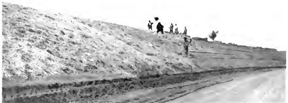
Spreading straw over top soiled slope to provide a mulch
